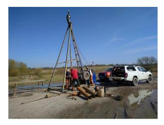
This may include sinking boreholes and trial pits, soil contamination testing, testing of coal tar macadam surfacing, ground gas and groundwater level monitoring, groundwater contamination, investigation of potentially worked coal seams (Coal Authority), and an initial geotechnical assessment of the ground conditions for foundation design.
