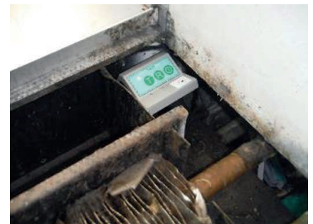
Fig 3: GT sensor mounted on bracket
