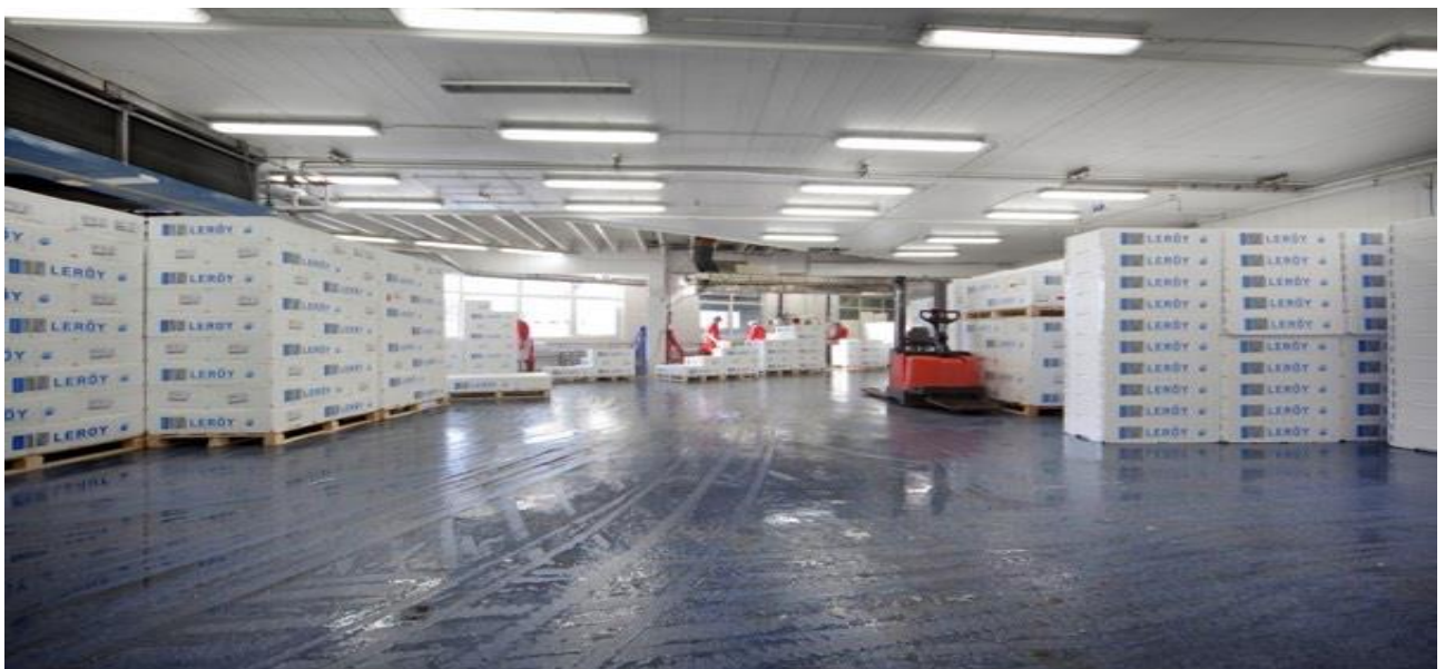
AcryliCon Décor System installed in 2004, Austevoll Fiskeindustri AS in Norway, Picture taken in 2010.
