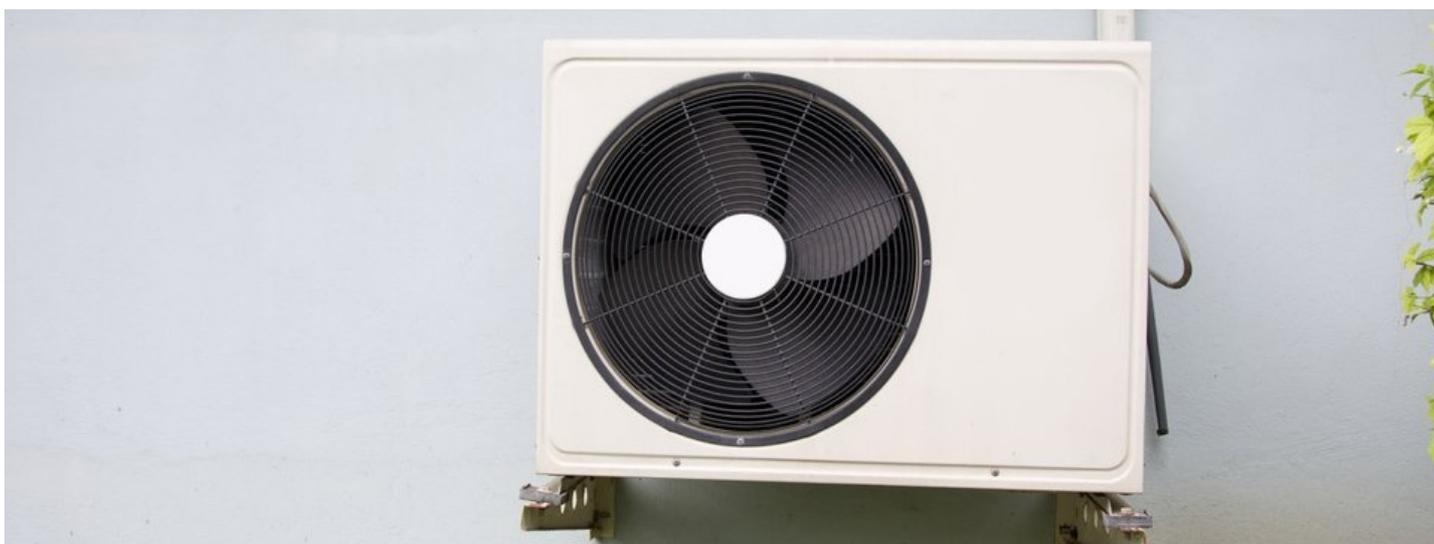
The energy performance of a heat pump can be determined according to the NTA 8800, which is based on the European standards EN 16147 and EN 14825/EN 14511. The efficiency of the heat pump will be expressed in terms of the coefficient of performance (COP). The COP relates the amount of heat that a heat pump emits to the energy used for it.
